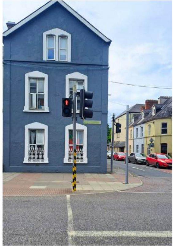
At The Traffic Lights, Cross to Mardyke Street
